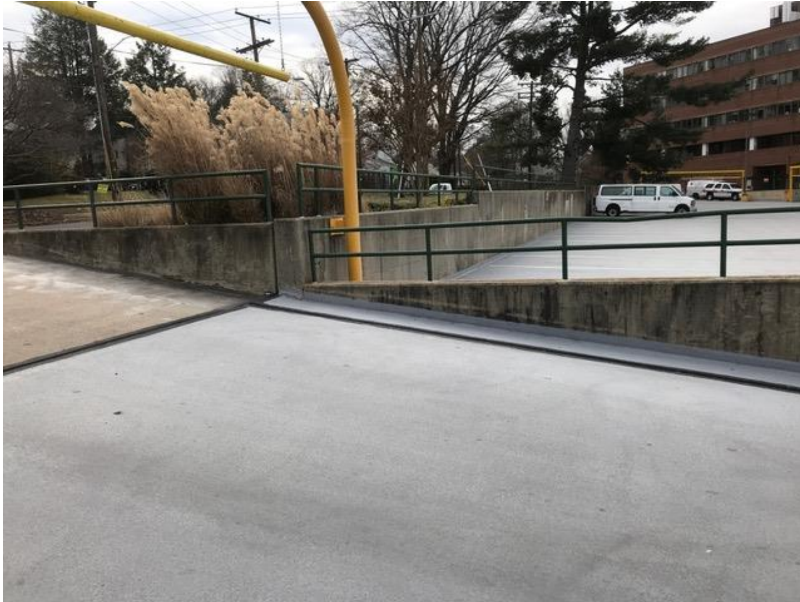
48 th Street Embankment
