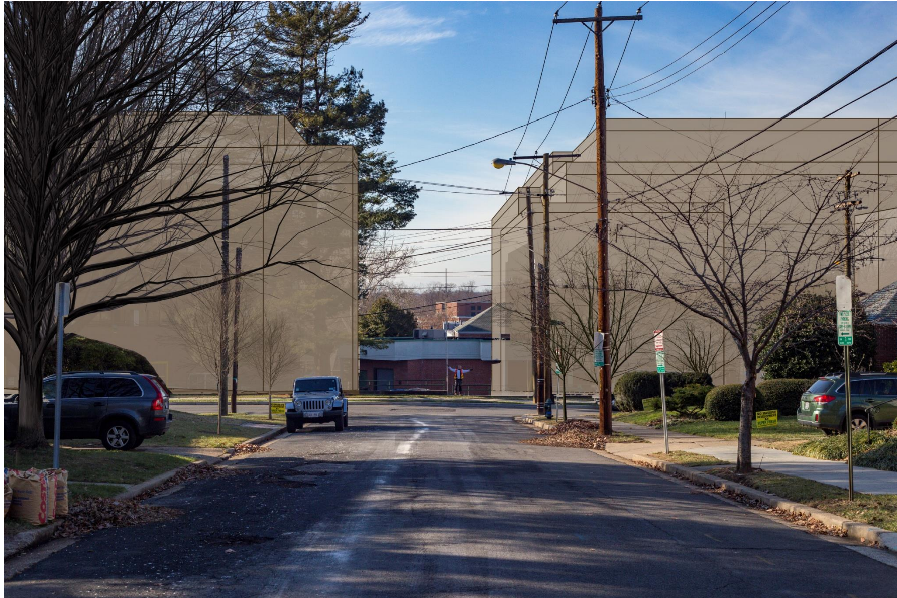
12-21-2017 Design as seen from Camera Loc. 01. The 3D model-massing accurately represents the height and width of the proposed development from this Windom Pl perspective. A 25ft tall survey rod is held by surveyor.
