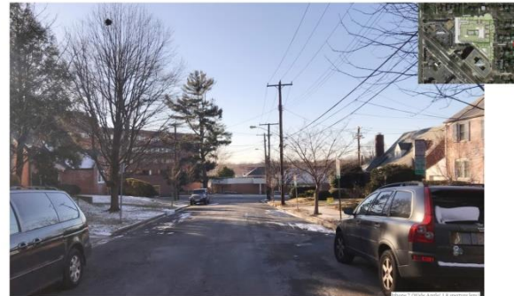
View from East - Existing (Window Place NW) VALOR DEVELOPMENT TORREY GALLAS URBAN A17 THE LADY BIRD
